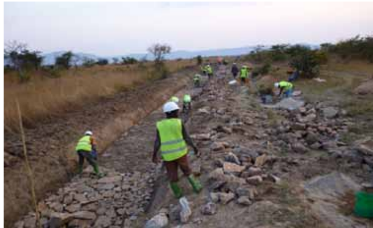
Figure 4.2: The Ongoing Construction Work Mbebe Irrigation Scheme
