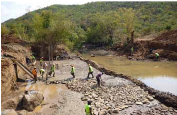
Figure 4.1: Ongoing Construction of the Ilulu Irrigation Scheme at Ikombe River Itumba
